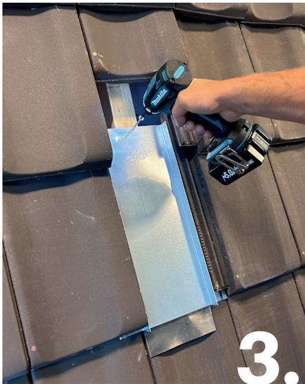
3. Secure metal tiles to roof battens using sealing screws.
